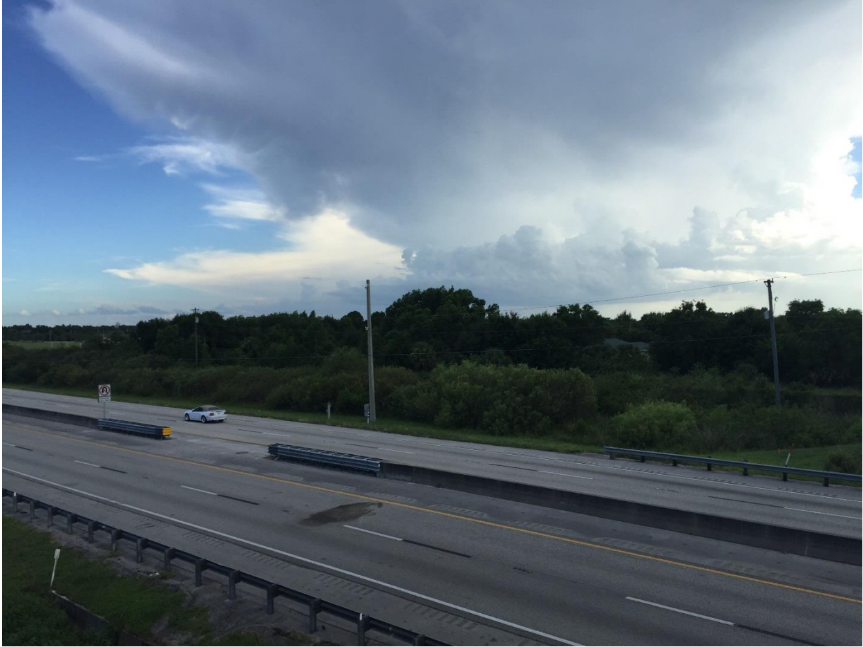
On Florida's Turnpike Overpass Facing Southwest
